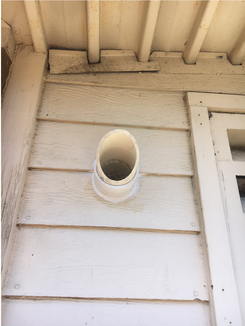
Vent pipe exiting the southern gable end of the building
